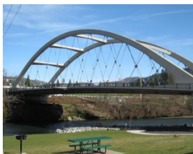
Depot Street Bridge at John F. Flemming Memorial Park
