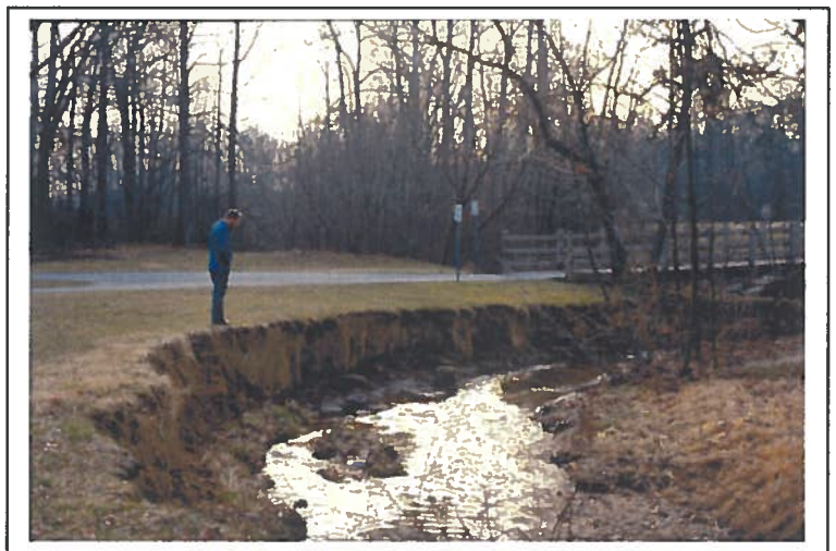
Figure 1-1(b): Stream downcutting resulting from stormwater runoff (Center for Watershed Protection 1999).
